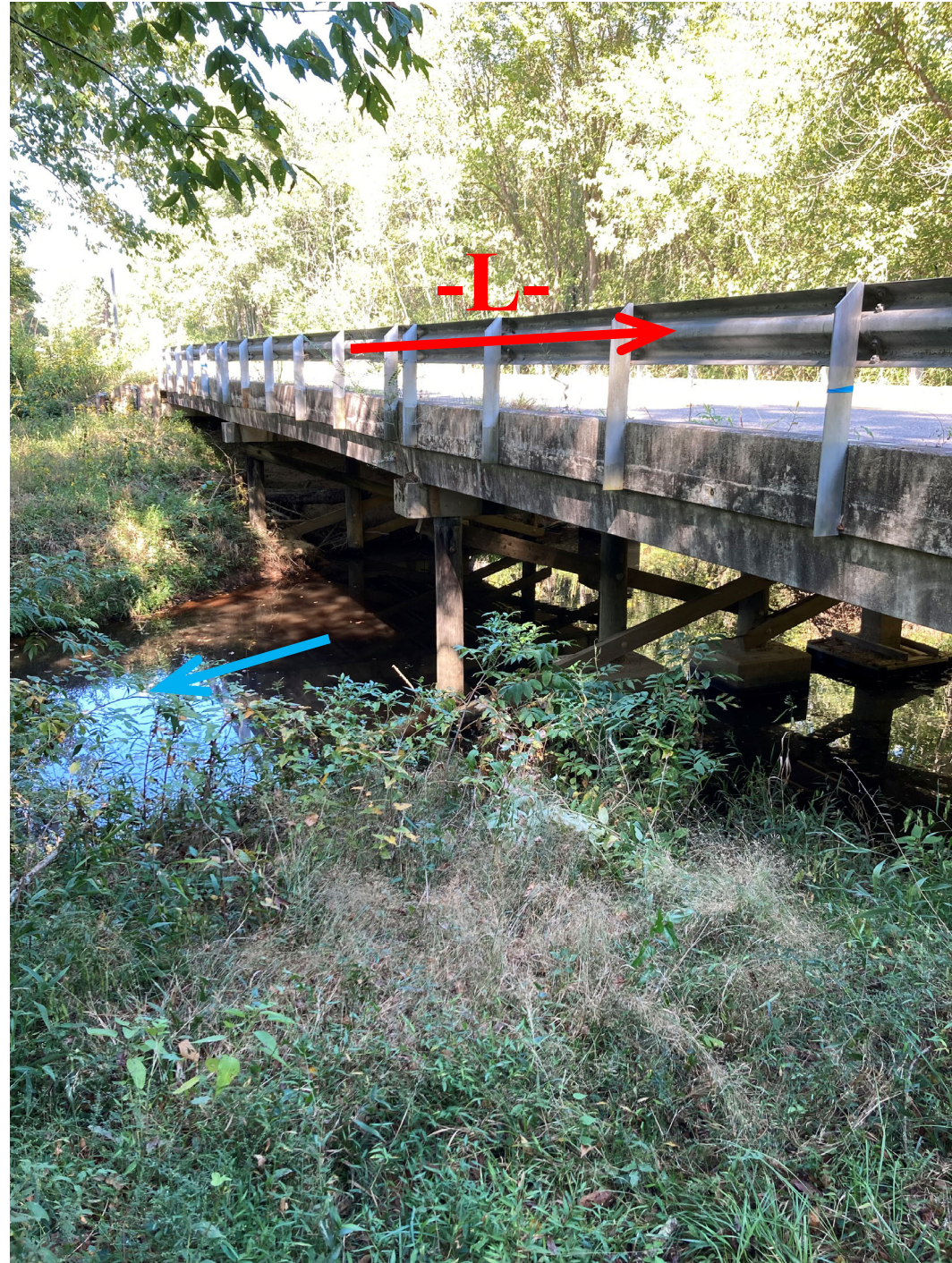
Looking Northwest towards End Bent 1
